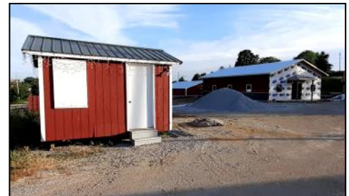
The old Santa House, in foreground, will be replaced by a much larger building allowing visitors to come in from the weather to greet Santa during Festival of Lights.
